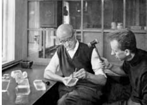
FIGURE 4 TECHNICIANS SPLITTING ICELAND SPAR CRYSTALS DOWN INTO PRISMS TO USE THEM IN OPTICAL DEVICES, PICTURE PROBABLY TAKEN IN THE BEGINNING OF THE 20TH CENTURY. HALLE, 1963.
